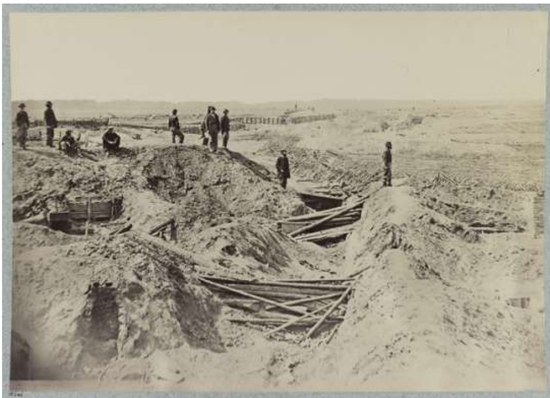
Picture of “Fort Damnation” taken April 3 rd 1865 showing Bomb Proofs with no breastworks or traverses on the left side of the picture indicating that is a picture of the rear of Fort Mahone that was unfortified. (damage seen most likely caused by the Confederate Artillery)
